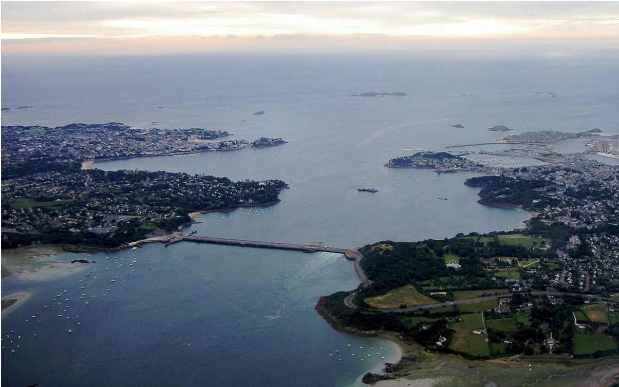
Figure 2-38: The Rance Tidal Power Station in France. [67] License: Public Domain
