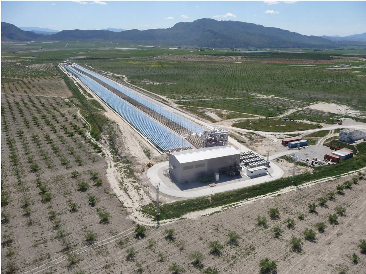
Figure 1-17: Linear Fresnel reflector technology at Puerto Errado 1 solar thermal power plant, Spain. [20] Licensed under Free Art License
