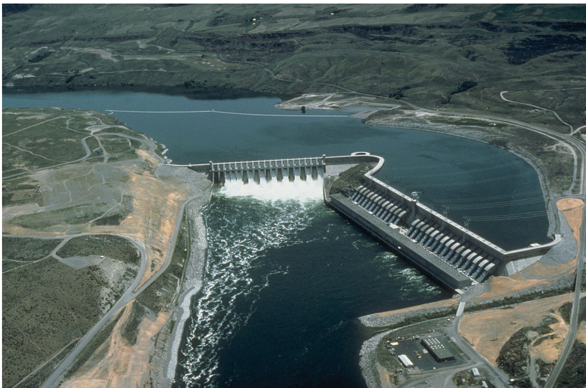
Figure 2-25: Chief Joseph Dam, a run-of-the-river plant in Washington, USA. [58] License: Public Domain
