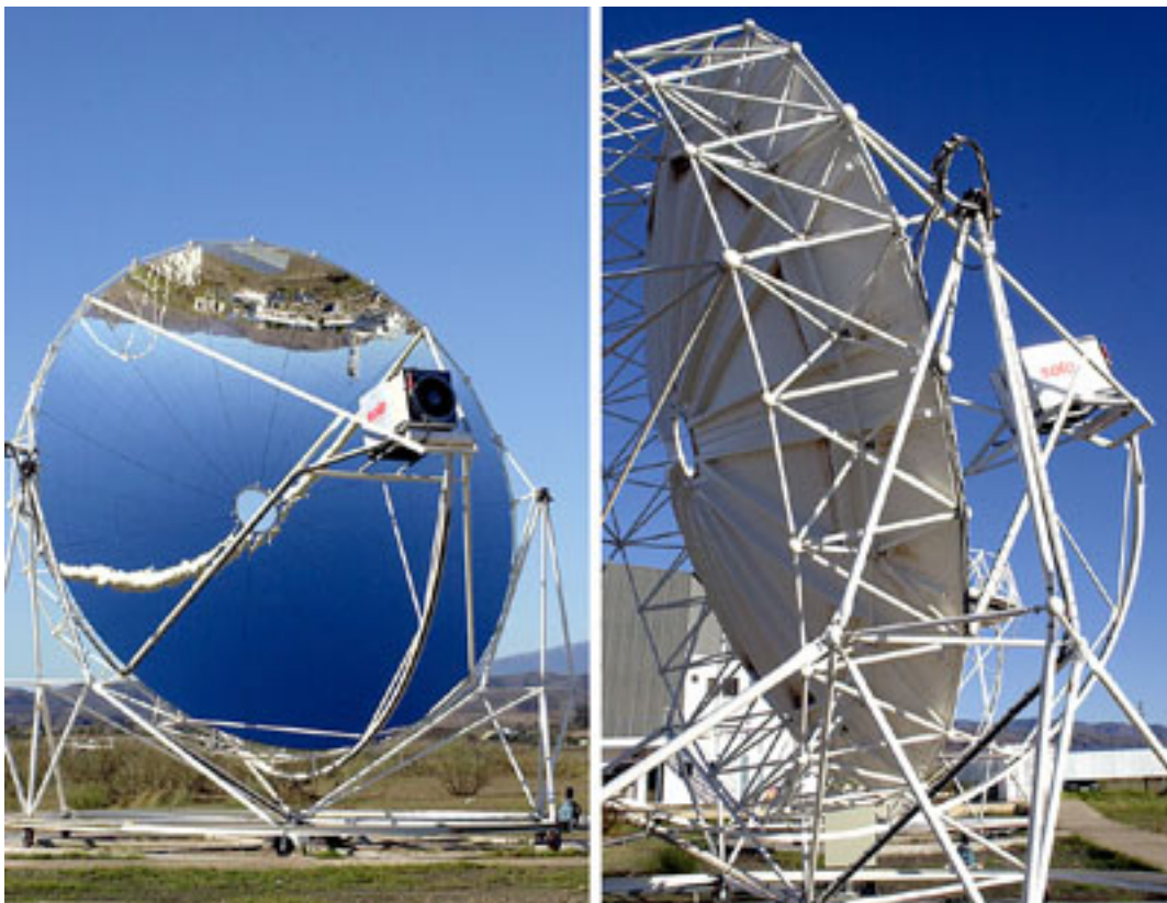
Figure 6-8: Dish Stirling system. [21]
