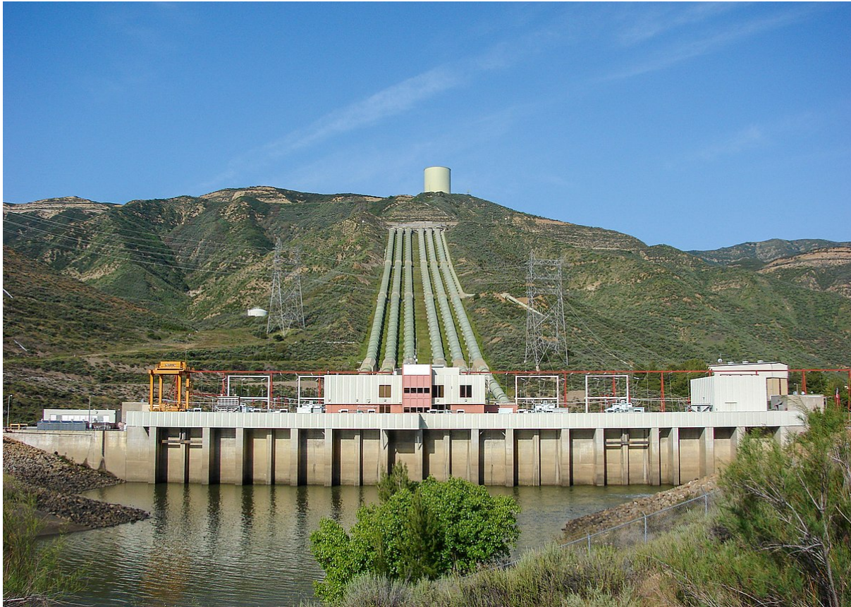
Figure 2-23: The Castaic Pumped Storage Plant, USA. [56] Licensed under CC BY-SA 3.0
