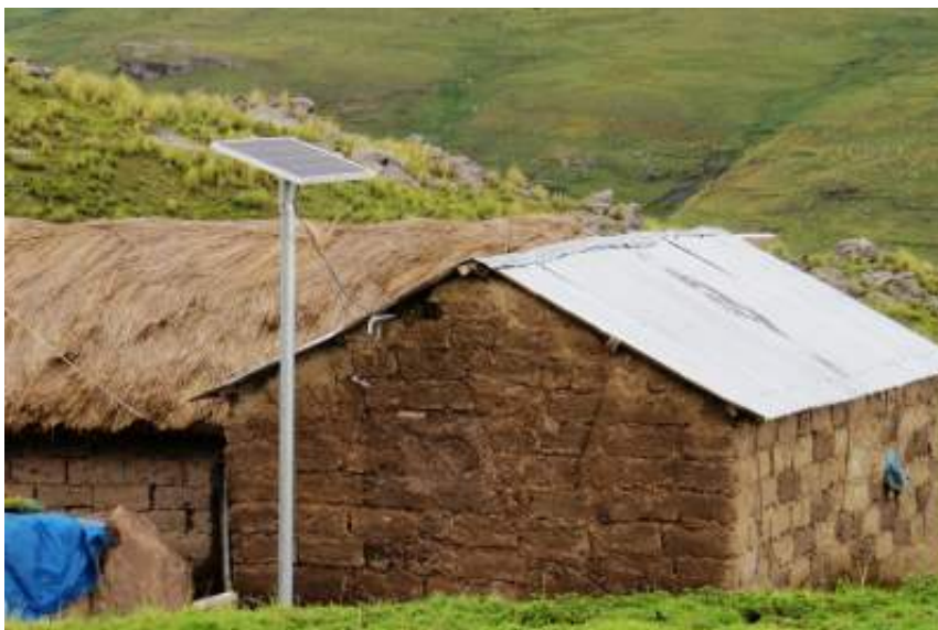
Figure 5-1: Solar home system in a house in Peru. [121] Licensed under CC BY-SA 3.0
