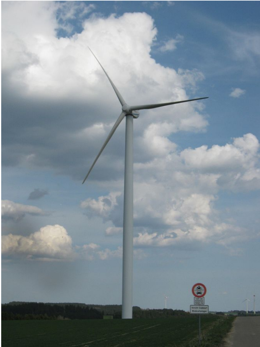
Figure 1-27: Horizontal axis wind turbine. [26] Licensed under CC BY-SA 3.0
