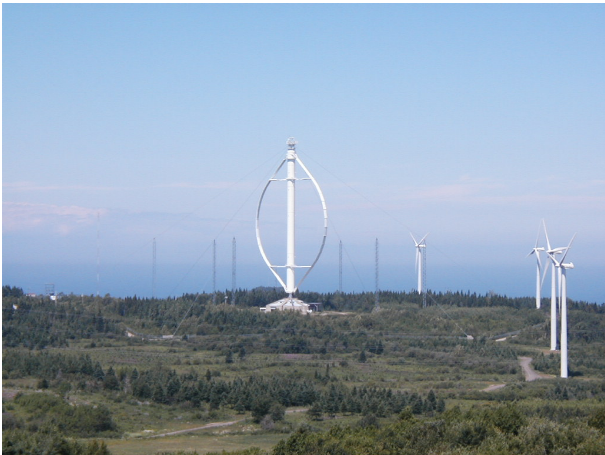
Figure 1-28: Darrieus wind turbine. [27] Licensed under CC BY-SA 3.0
