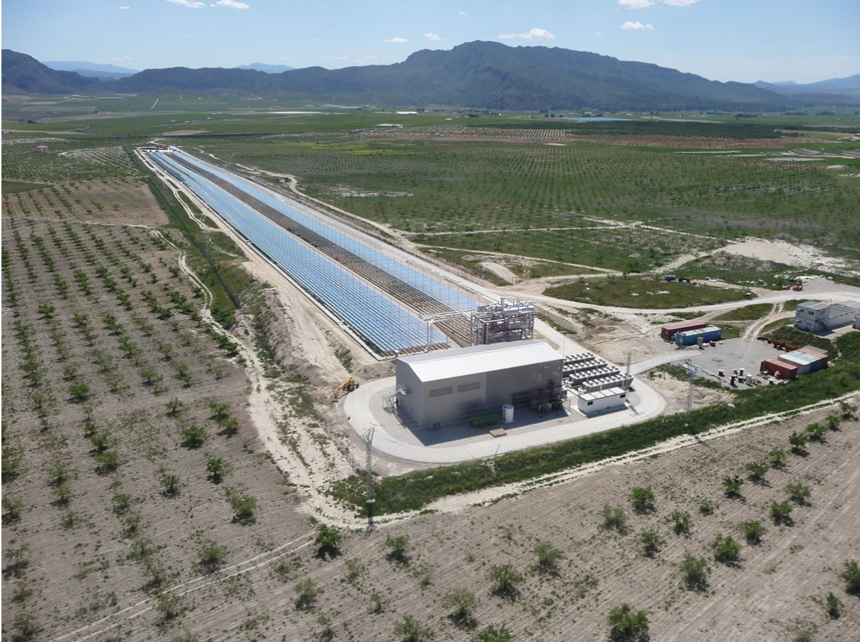
Figure 6-5: Linear Fresnel reflectors. [20] Licensed under Free Art License
