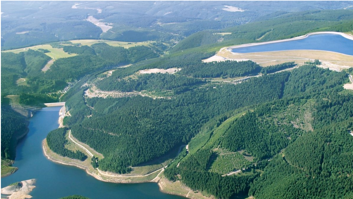
Figure 11-17: Goldisthal Pumped Storage Hydro Electric Dam in Germany (Credit: Voith under Written Permission, [398])
