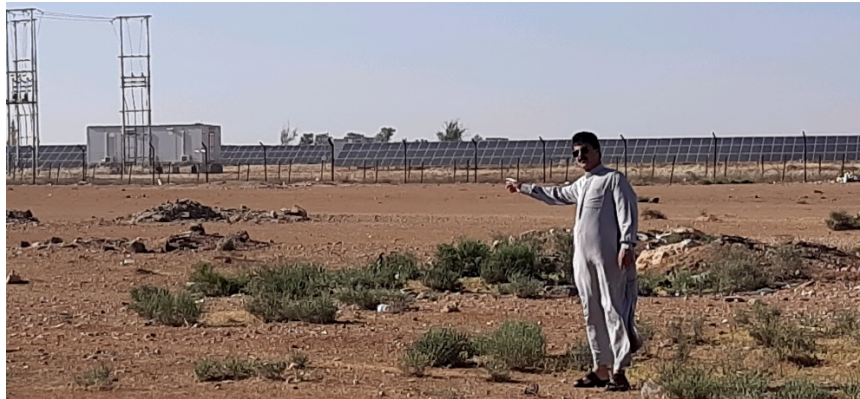
Figure 12-8: Mega solar system to supply main grid
