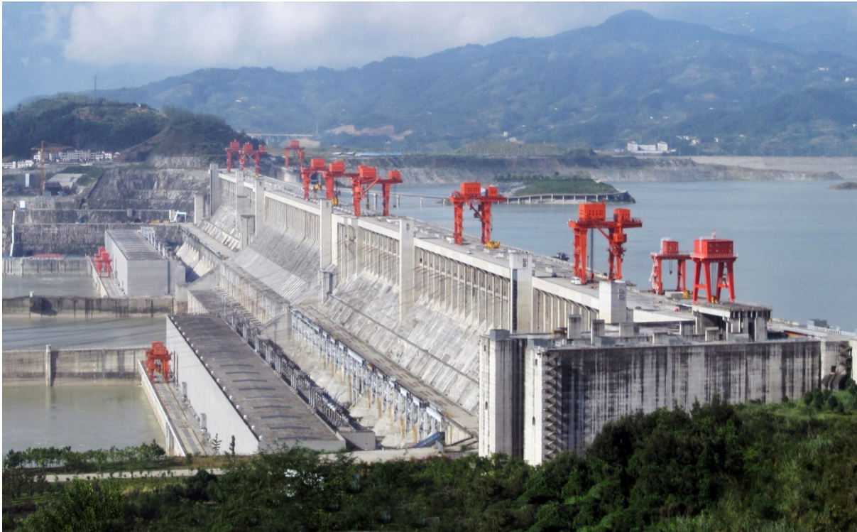
Figure 11-16: Three Gorges Hydro Electric Dam in China (Credit: Le Grand Portage licenced under CC BY 2.0, [52])
