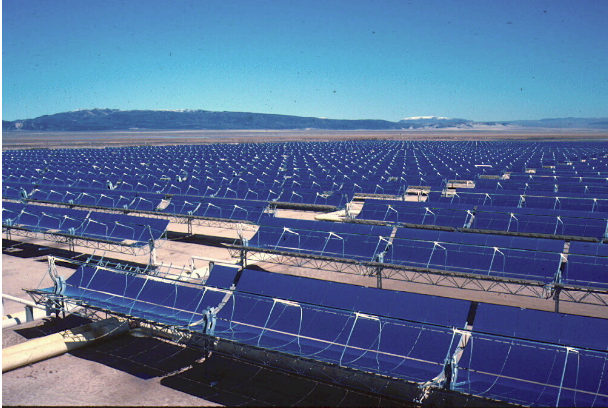
Figure 6-3: Parabolic troughs. [19] License: Public Domain
